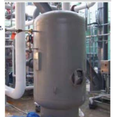
(1) Recirculation Pump Skid (1) Backwash Air Receiver
